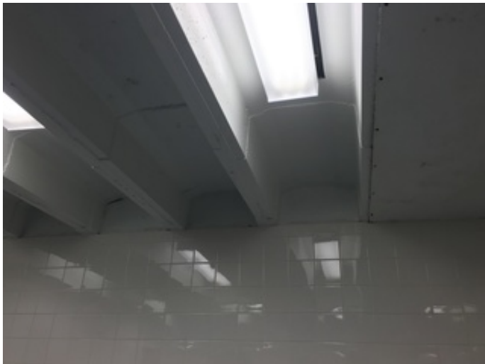
Pre-fab concrete deck
