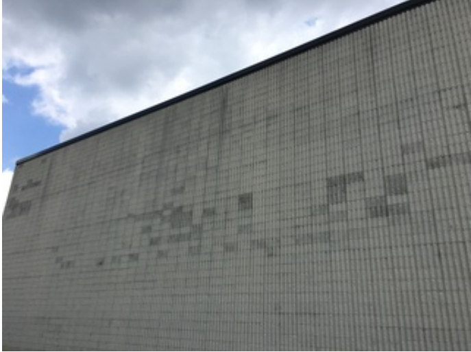
Typical CMU wall
